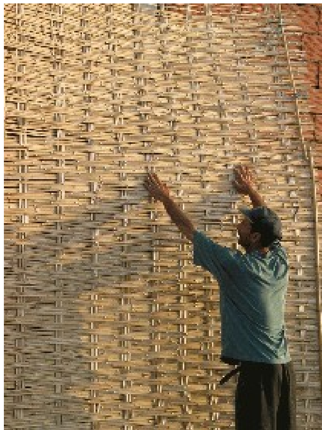
Abdil Nabi, the qassab, weaving one of the three 5.50x2.08 M reed mattes used in covering the newly construction vault (Photo: A. el-Habashi)
