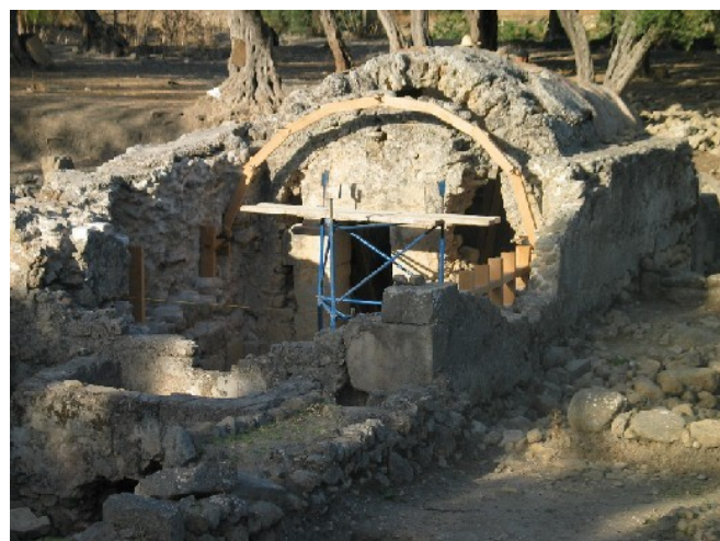
Left: Design of assemblage joints between posts, wooden tie, and frame members (by A. el-Habashi); Right: the erection of the first wooden frame at the west of room 5. 4
