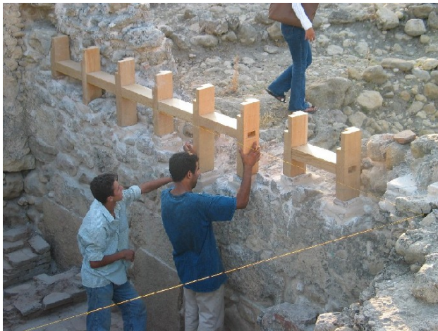
Left: The carpenter and his assistant fixing the posts directly on the ruined walls. Note the different height of the posts to compensate the uneven profile of the ruined walls (A. el-Habashi);
